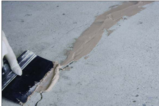
Example: Patching cracks, pits & divots
