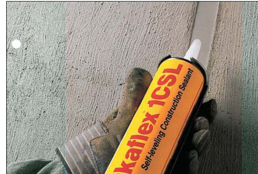
Example: Filling expansion joints
