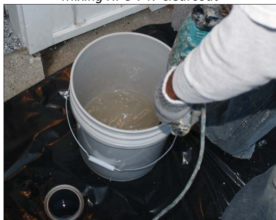
Mixing HPU 747 clearcoat
