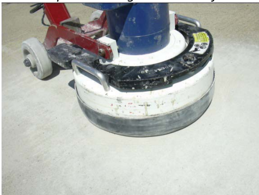
Example: Grinding concrete surface
