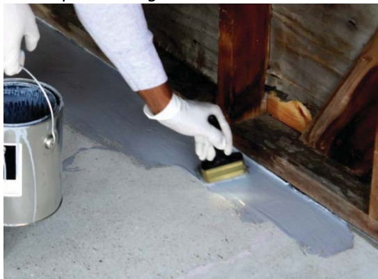
Example: Cutting-in Norklad WB basecoat
