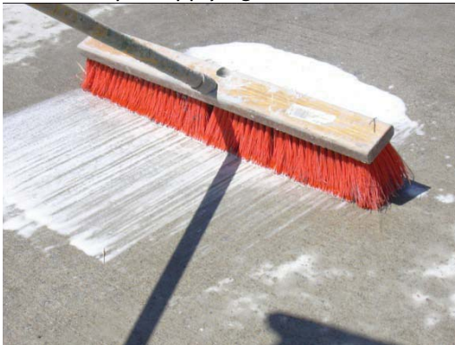
Example: Applying Etch N' Clean
