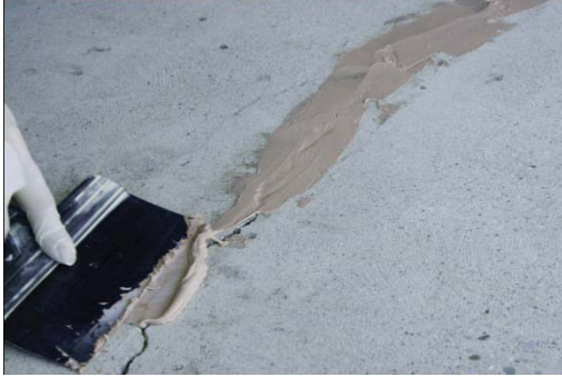
Example: Patching cracks, pits & divots
