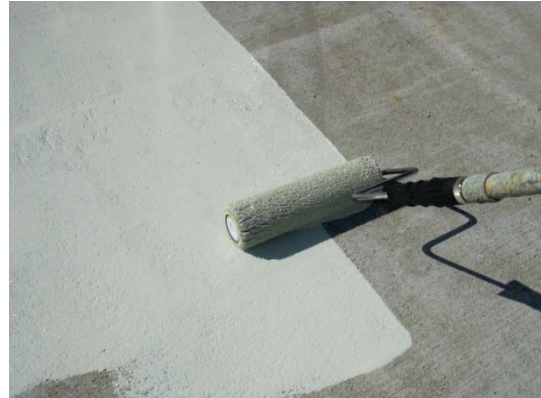
Example: Roller applying Norklad WB Basecoat
