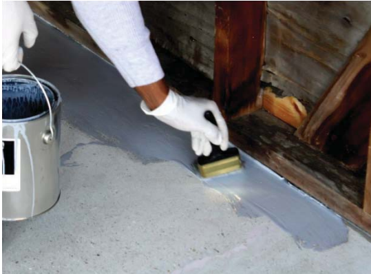
Example: Cutting-in Norklad WB basecoat
