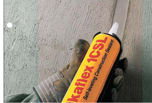
Example: Filling expansion joints
