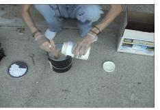
Be sure to roll one even coat of Crystal Clear topcoat to entire surface to be coated (we recommend a good 3/8" nap roller). Material will go on as a milky white (may even look like white paint) and dry Crystal Clear. Smooth out any visible clumps of clear coat. If you come to the end of your floor and you still have clear coat left over do not use the mixed
