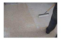
**Dry Time: Dries to light foot traffic on concrete floors in 24-48 hours.** You can move heavy items on it in 36-48 hours. **Full cure for vehicle traffic in seven days.** Low temperature, high humidity, thick films or poor ventilation will increase these times. Lack of ventilation and/or the use of portable fuel burning heaters that produce exhaust gases, during
